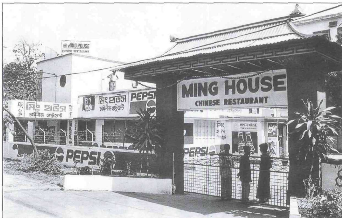
Early in the 1970s the UNICEF Bangladesh office moved to this building on Mirpur Road in Dhaka — now, in 1995, the "Ming House" chinese restaurant.
