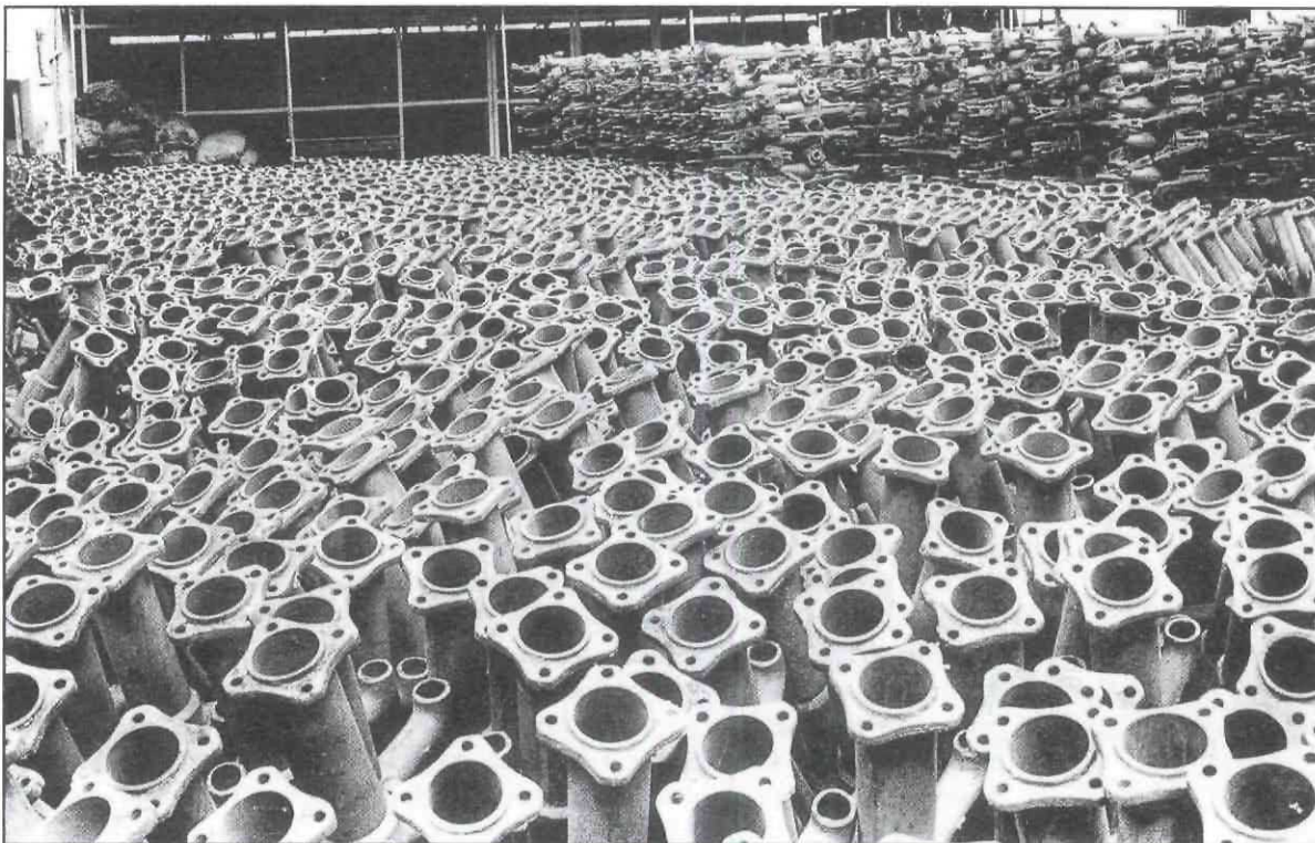
No. 6 Suction Pumps, in a DPHE yard in the early 1970s, awaiting distribution.
